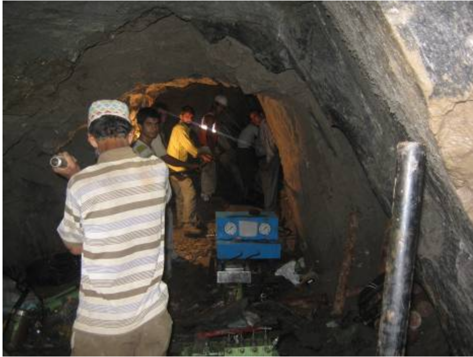
Fig. 8: Preparatory Work for Hydraulic Fracturing Test in Horizontal Bore Hole
