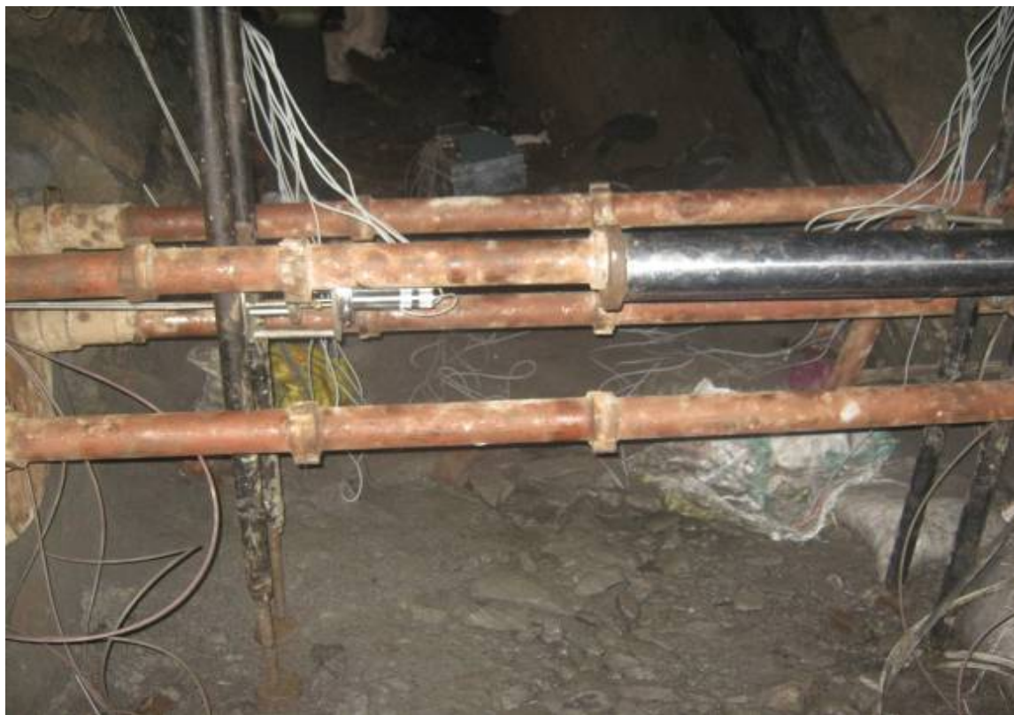
Photograph 1: Typical Plate Jacking Test Set Up (Horizontal Direction) in Drift
