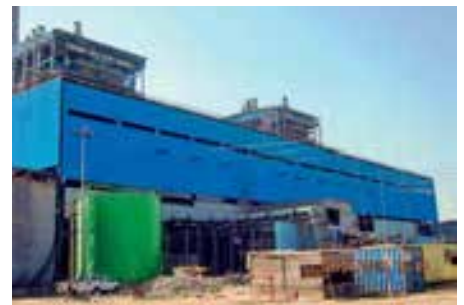
Main Power House
