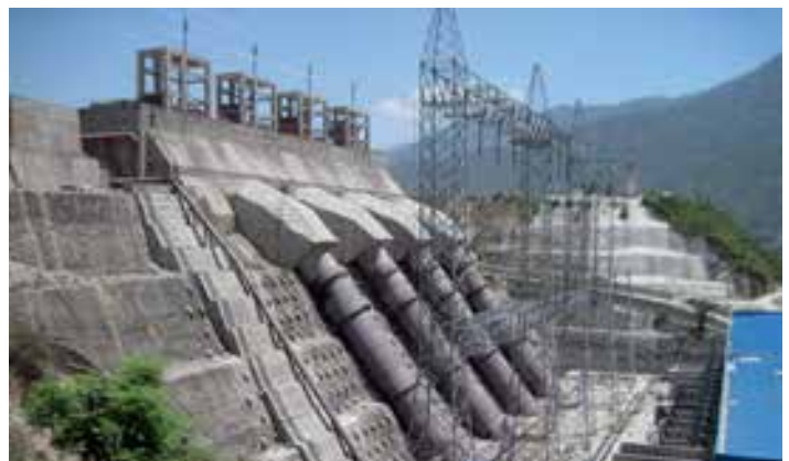
Penstocks view at the Power Station
