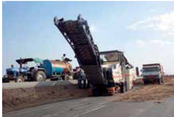
Milling Machine correcting the surface of existing road
