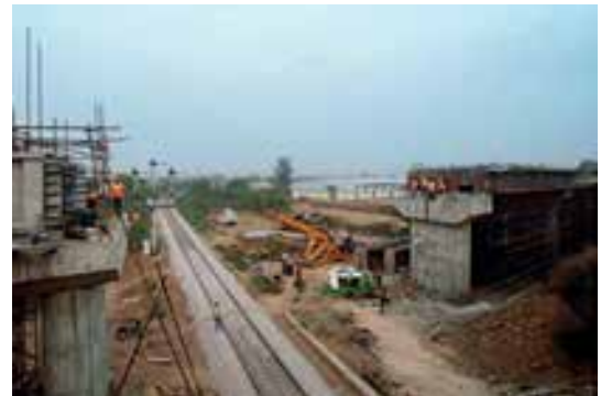
Rail Over Bridge under construction
