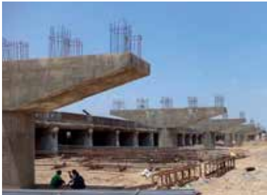
Construction of pier caps complete
