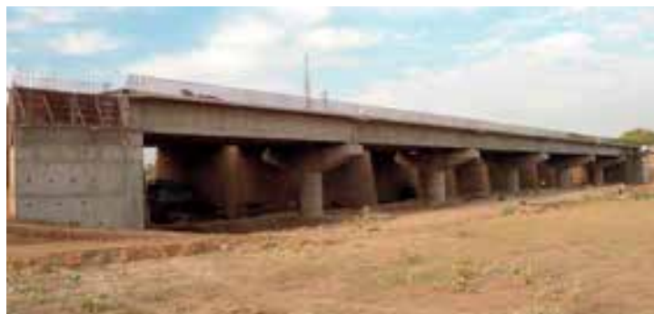
Construction of Deck Slab on the on-bridge complete
