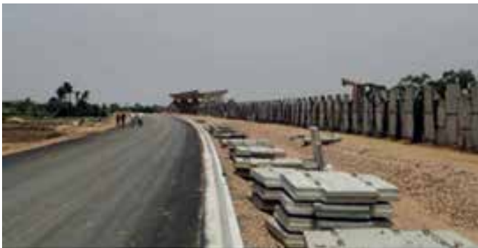
Re-Wall Kota End work in progress
