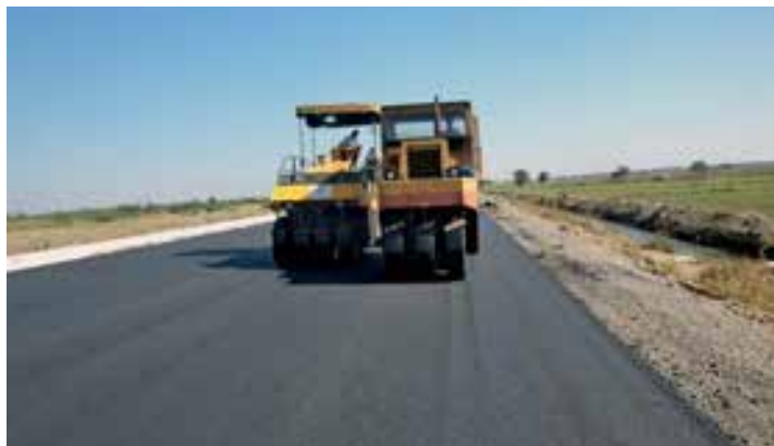
Road-top laying in progress at Bagodara Vasad Expressway
