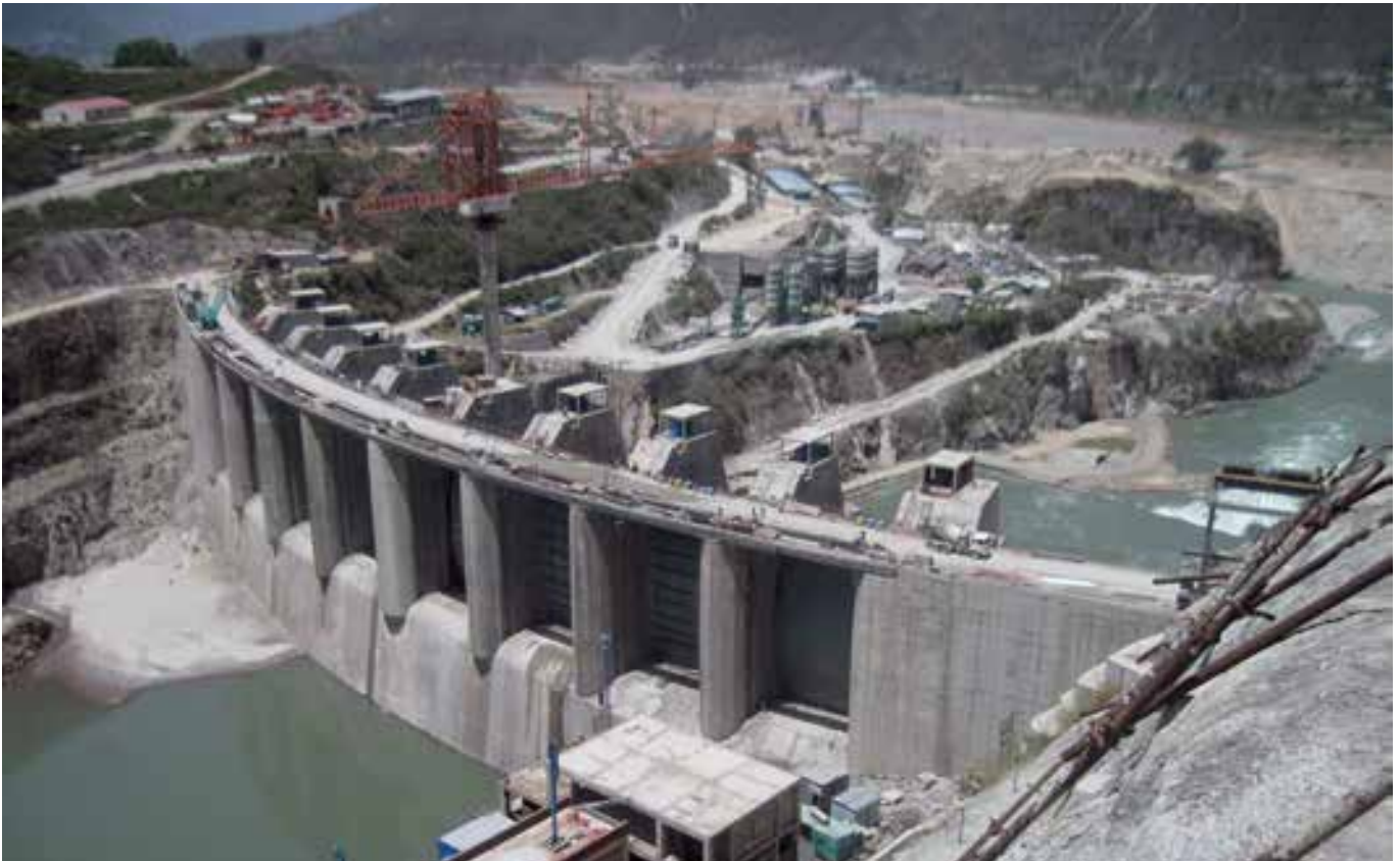
Upstream radial view of dam
