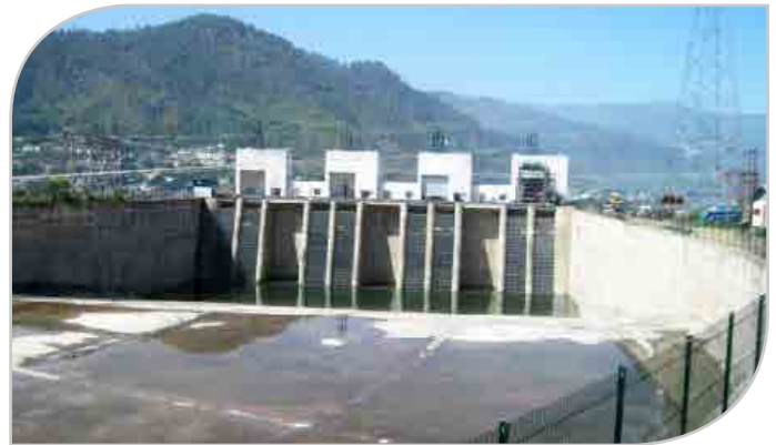
Forebay Intake Structure
