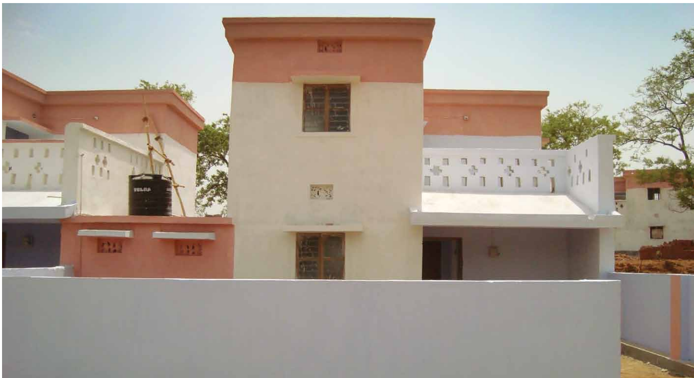
Construction site of R & R (Rehabilitation & Resettlement) colony for Project Affected Families (PAF) in Tokisud Coal Mines, Jharkhand.
