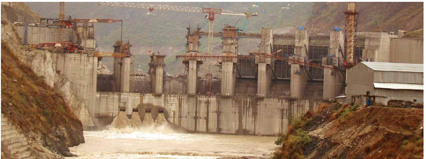
A view from the downstream side of the dam structure at Shrinagar Hydro Electric Power Project.
