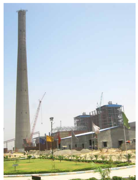
Standing Tall: A 275 m high chimney of Goindwal Sahib Power Plant.
