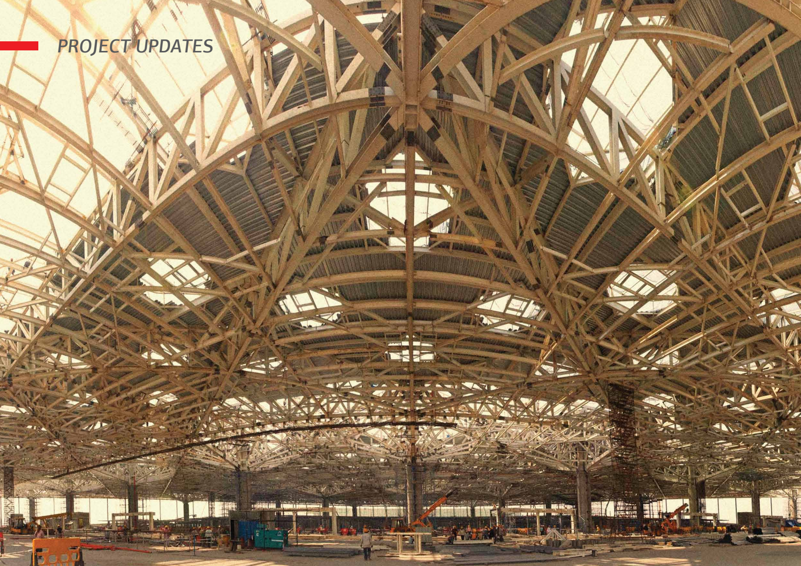
The mega roof closure work in progress at T2
