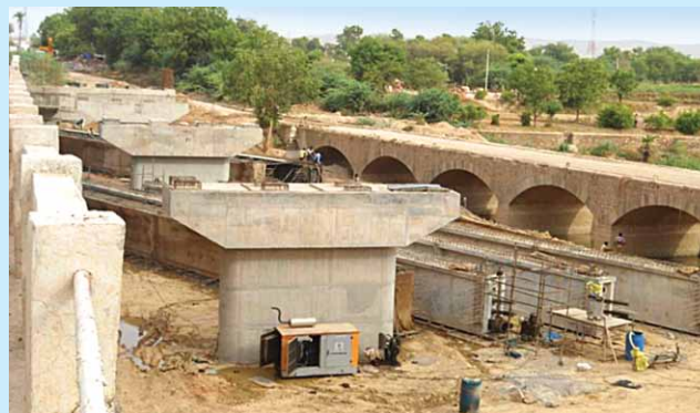
Girder casting under progress (Deoli-Kota Expressway)
