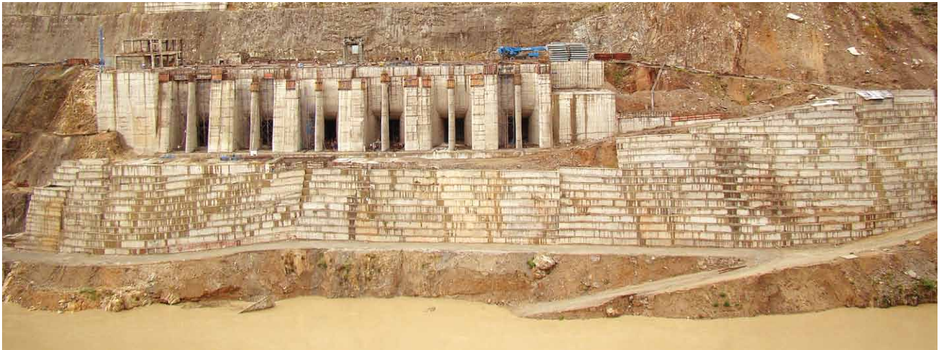
Closer view of Head Race Tunnel intake structure being built on RHS flank at Shrinagar Hydro Electric Power Project
