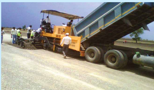
Work in progress at Bagodara – Vasad Road Project.
