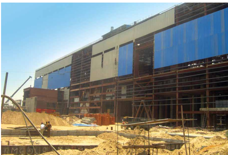
Transformer yard and power house building at 2x270 MW Goindwal Sahib Thermal Power Project, Punjab.
