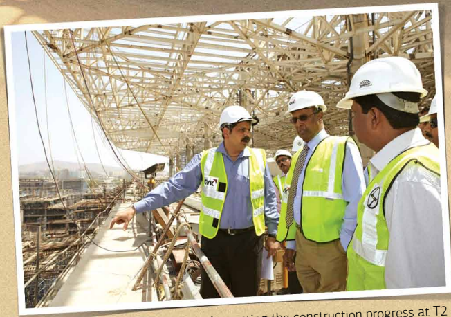
Chairman inspecting the construction progress at T2
